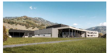
What WITTENSTEIN AG in Grüşch will look like after the expansion.
